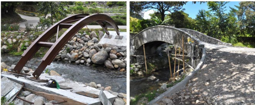
Construction of the "Grande" Bridge (Made of Cement).
